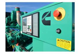
**Warning:** Backfeed to a utility system can cause electrocution and/or property damage. Do not connect GenSets to any building electrical system except through an approved device or after the building main disconnect is open. Neutral connection must be bonded in accordance with National Electrical Code.
