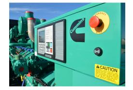
**Warning:** Backfeed to a utility system can cause electrocution and/or property damage. Do not connect GenSets to any building electrical system except through an approved device or after the building main disconnect is open. Neutral connection must be bonded in accordance with National Electrical Code.
